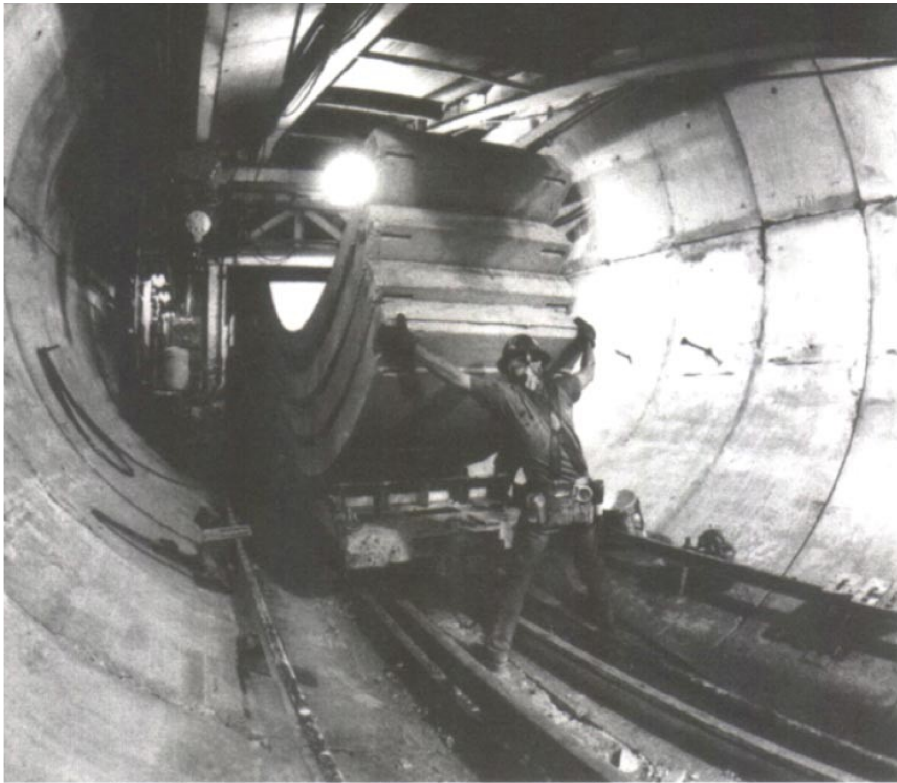
Worker installing concrete tunnel linings. Photo courtesy of MTA
