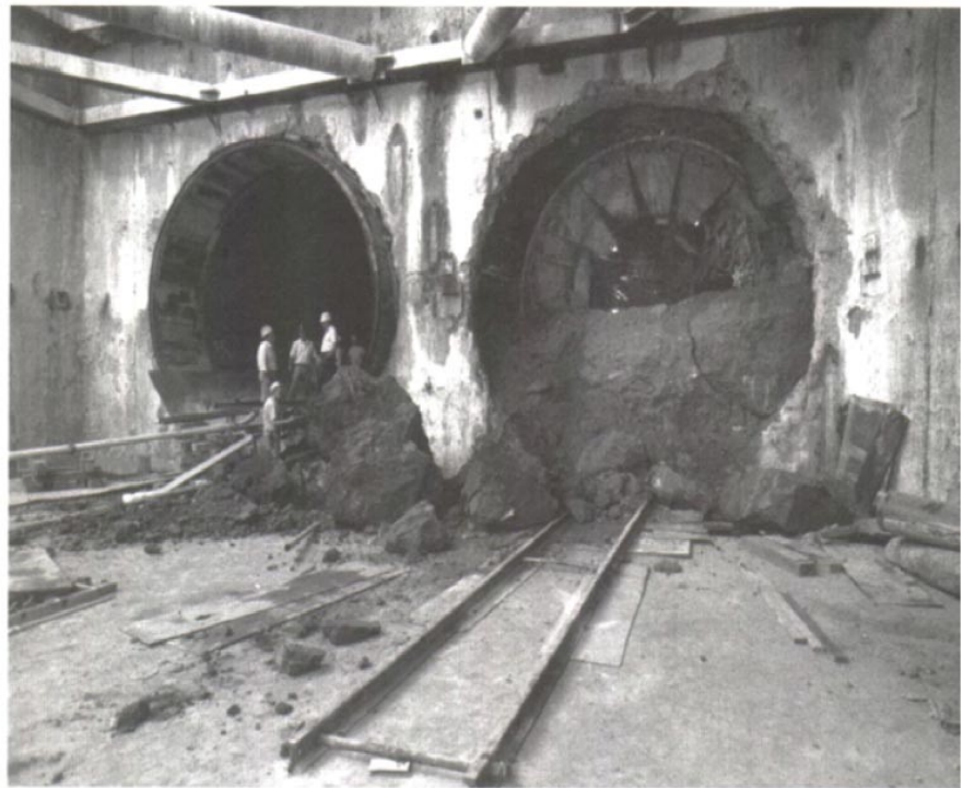
Tunnel breakthrough, Red Line subway. Photo courtesy of MTA
